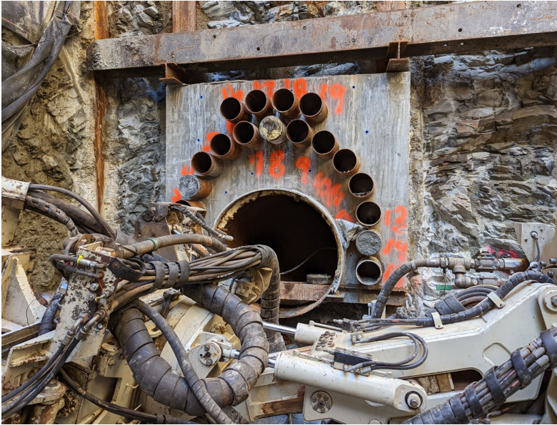
Horizontal Pile (Spile) installation (Top left)
