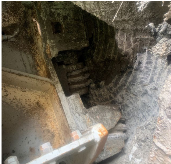
Horizontal Pile (Spile) installation (Top left)
